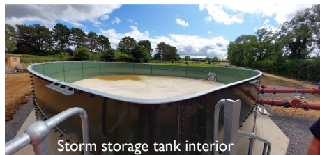
Storm storage tank interior
